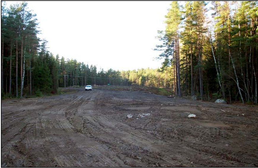
Figure 9.3. Photograph towards the east after the completion of the cover Photo: M. Bäckström
