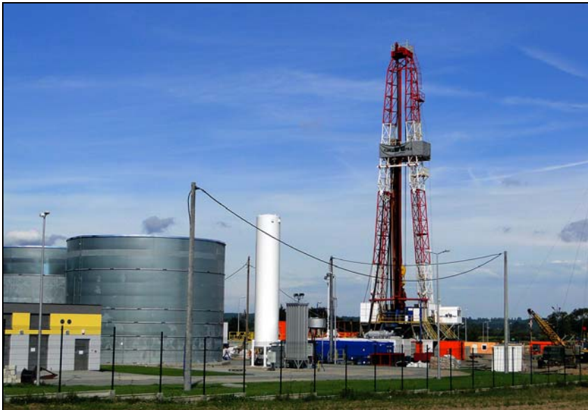
Figure 6.27. Building site of the Kosakowo Underground Gas Cavern Storage; Poland
