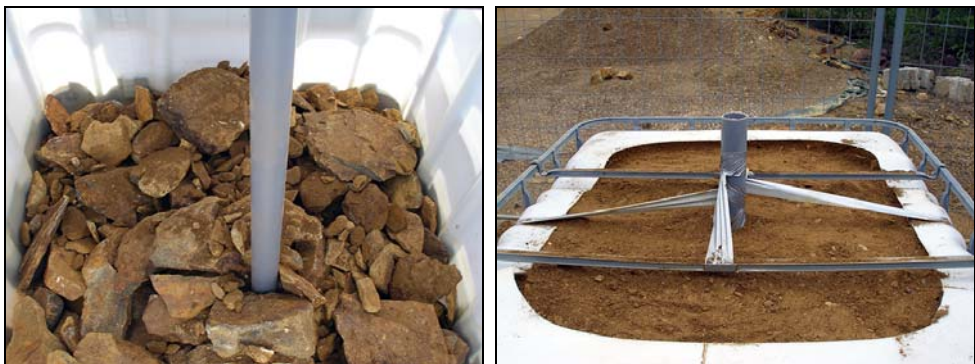
Figure 9.1. Pilot scale trials 1 m 3 during construction (left) and after completion (right)
