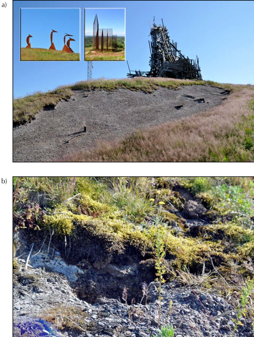
Figure 9.8. Kvantorp mining and processing waste dumps in Sweden: a) artistic installation and small landslide, b) burning part of waste dump
