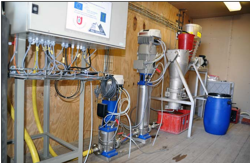
Figure 3.15. Mobile pilot unit for element extraction and recovery Photo: A. Ostrega
