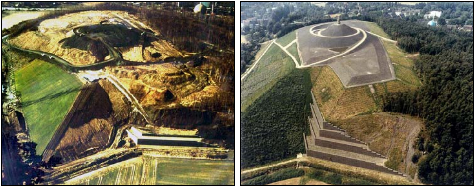
Figure 9.7. Rheinebble waste dump at a hard coal mine in the German Ruhr Area: (left) during reprofiling process, (right) after regeneration secured by gabion wall and equipped with artistic element “Stairways to Heaven”
